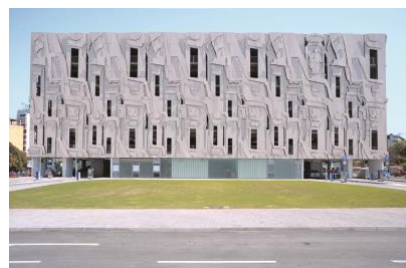
Façade, Parking house Skopje, Northern Macedonia, 2013. © Darko Hristov
