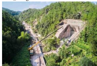
Baustelle Quarry #10, Foto: Wang Ziling © DnA_Design and Architecture
