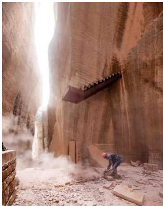
Baustelle Quarry #8, Foto: Wang Ziling © DnA_Design and Architecture
