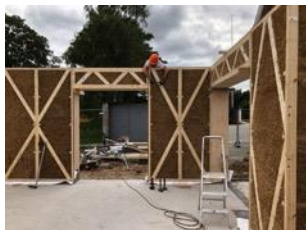
Straw Construction © Henning Larsen Feldballe School is built up of wooden elements of straw that doubles as insulation and structure of the building.
