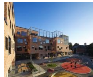
Frederiksberg School © Hufton+Crow Reused bricks not only influence a building's appearance and identity, they also have a huge impact on the building's CO2 footprint compared to
