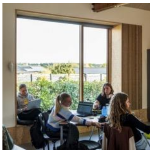
Feldballe School © Rasmus Hjortshøj - COAST Extension to Feldballe School built entirely out of straw, wood, seagrass and clay, Rønde, Denmark.
