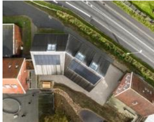
Feldballe School 2022 © Rasmus Hjortshøj – COAST In the small rural town of Rønde, located in the heart of Denmark, lies Feldballe School that is totally redefining the standards for sustainable construction.
