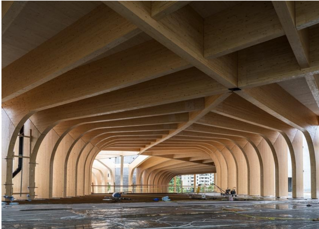
World of Volvo Construction site, June 2022 Photo: Rasmus Hjortshøj – COAST
