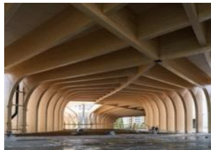
World of Volvo Construction site June 2022 © Rasmus Hjortshøj - COAST Designed around the Swedish concept of "Allemansrätten", denoting a fundamental right to nature or 'the freedom to roam', World of Volvo, a 20,500 m2 experience center in Gothenburg, will offer an open invitation to the public. The building uses a timber structure to embody the regional landscape in both form and materiality.
