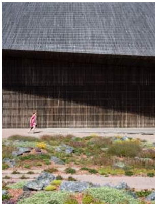
The Wadden Sea Centre, Esbjerg, Denmark. © Adam Mørk
