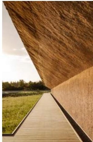
The Wadden Sea Centre, Esbjerg, Denmark. © Adam Mørk
