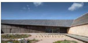
The Wadden Sea Centre, Esbjerg, Denmark. © Adam Mørk
