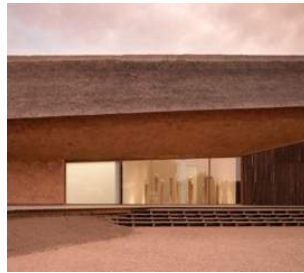
The Wadden Sea Centre, Esbjerg, Denmark. © Adam Mørk
