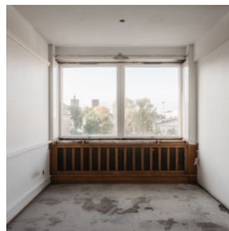
Kristian August Gate 13 in Oslo by Mad arkitekter; Office space before renovation. © Kyrre Sundal
