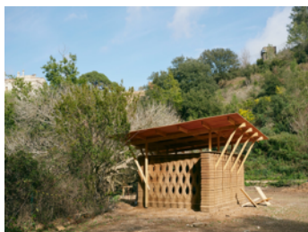
3D-printed earth housing prototype. © IAAC
