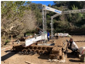
3D-printing of the earth prototype with WASP printer. © IAAC
