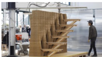
3D-printed earth wall with integrated timber stairs (1). © IAAC
