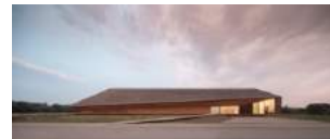
The Wadden Sea Centre, Esbjerg, Denmark. © Adam Mørk
