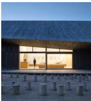
The Wadden Sea Centre, Esbjerg, Denmark. © Adam Mørk
