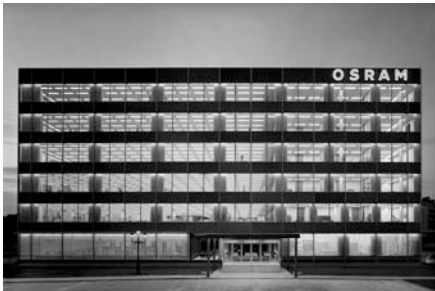
Osram Administration Building, 1966 © Heinrich Heidersberger
