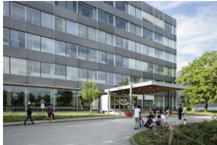
Osram Administration Building, 2016 © HGEsch
